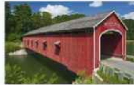
K505 Covered Bridge
